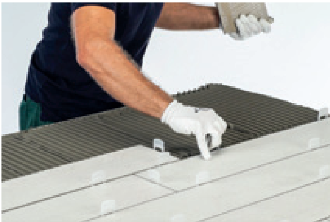
disposable clips installation
