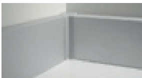
95/7I inside corner
